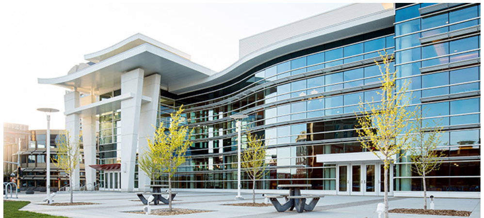
Union-built Mayo Civic Center Expansion in Rochester made the 2017 Finance & Commerce TOP PROJECTS list. (Photo by F&C News)
